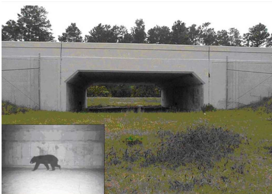
Prefabricated concrete box culvert along SR 46 in Seminole County, Florida. (Source: Wildlife Crossing Handbook Randy S. Kautz, Stephen R. Bittner, and Tom H. Logan)
