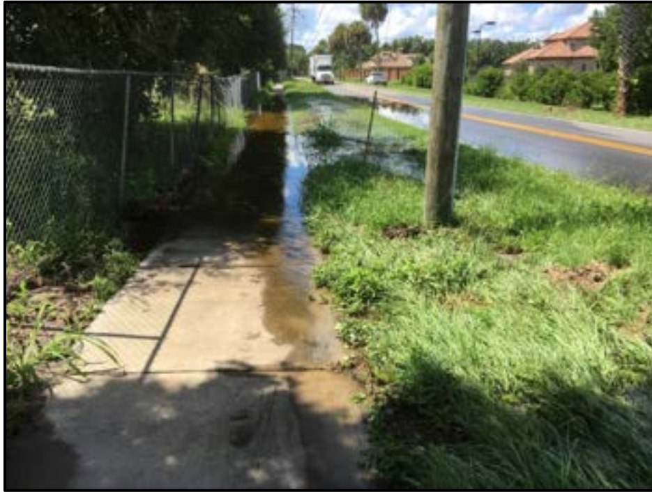
Photo 5 – View to south along Lake Markham Road, flooding in swale and into travel lane on east side of road (~900' north of Markham Road).
