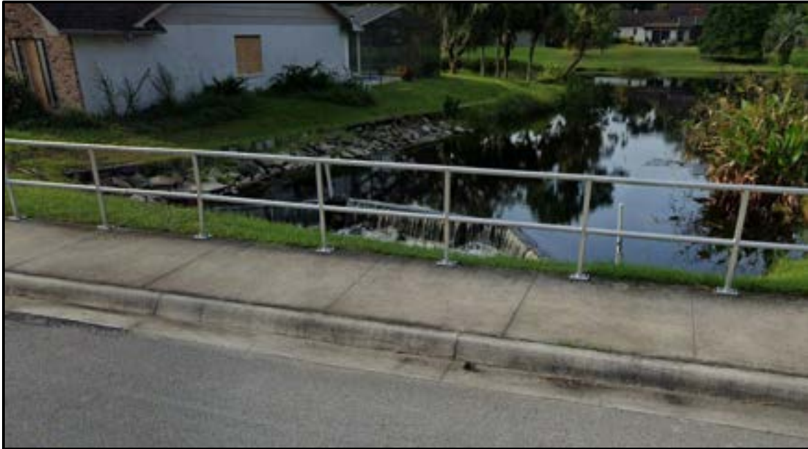
Photo 3: Stormwater Pond Outfall Weir Structure
