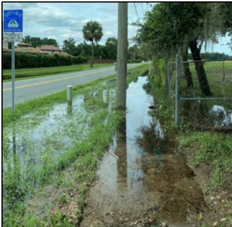
Photo 4 – View to north from the intersection of Lake Markham Road and Roberts Place Court – flooding in swale and sidewalk.
