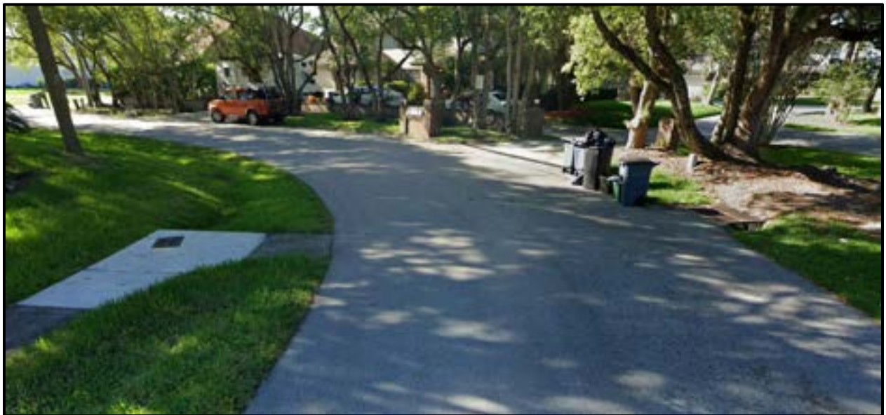
View to southeast along Cutler Drive towards at turn, note mismatched inlets, driveway trench drain, and undersized swales (Google, 2019)
