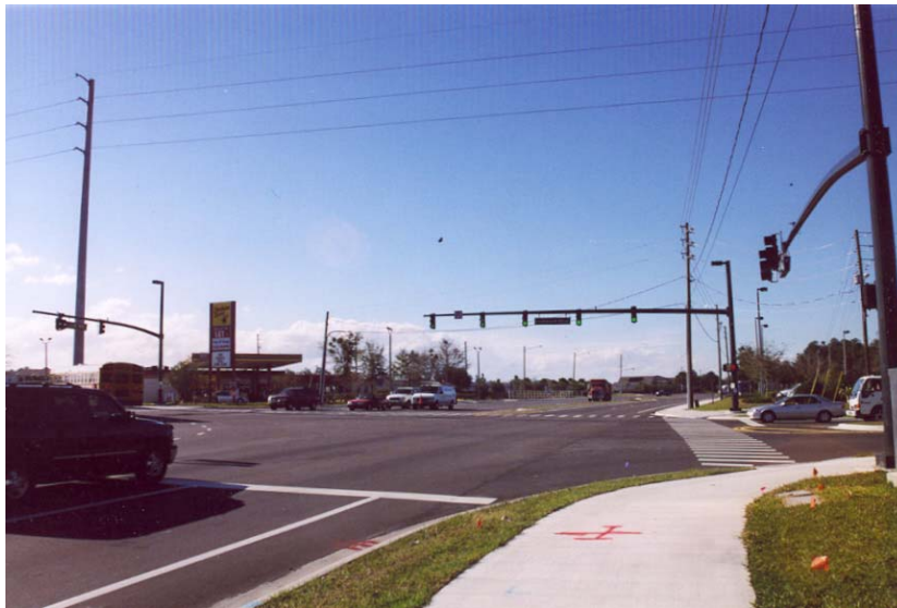
Intersection at Lockwood Boulevard and CR 419 showing improved commercial use adjacent to the project roadway.
