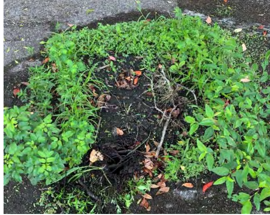
Fig. 4.9.7.B – Sedimentation Clogging Grate Inlet
