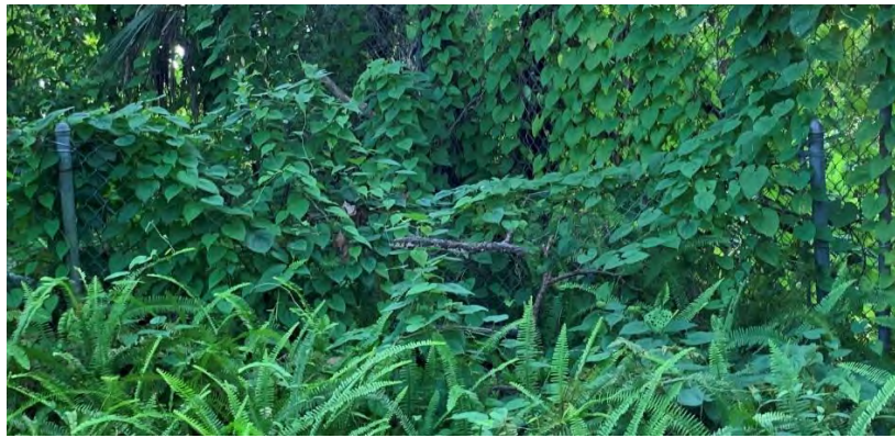
Fig. 4.9.6 Fence Impacted by Debris
