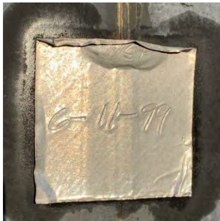
Fig. 4.9.5 Light Pole Date Data
