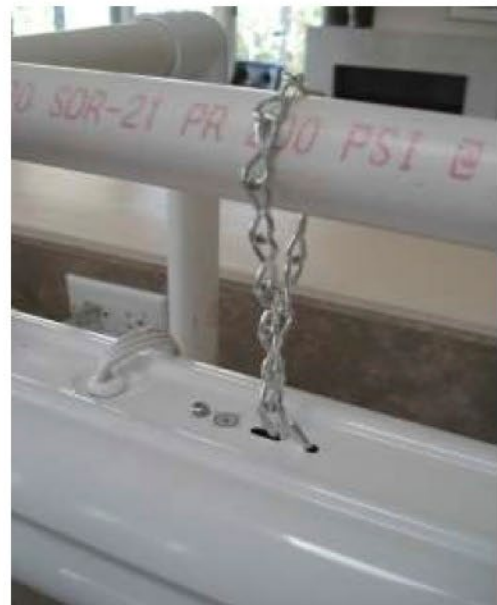
Figure 3 Detail of chain and "S" hook attachment
