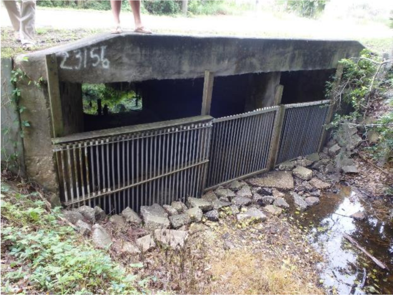
Photo: Mills Creek grass carp barrier.
