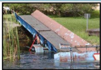
Harvesting Machine Being Set in Place
