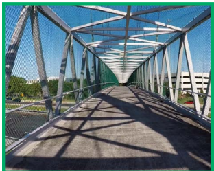
I-4/Cross Seminole Trail Bridge
