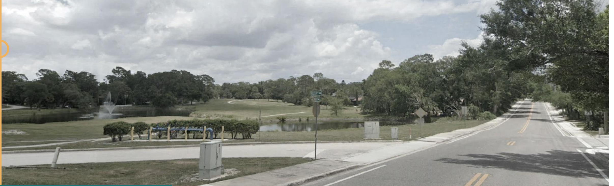
North Street Roundabout
