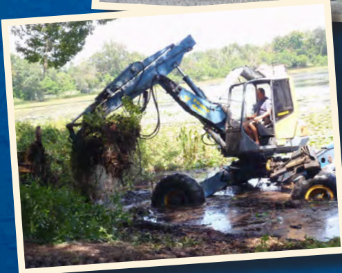
Roads-Stormwater Clears Clogged Retention Pond.
