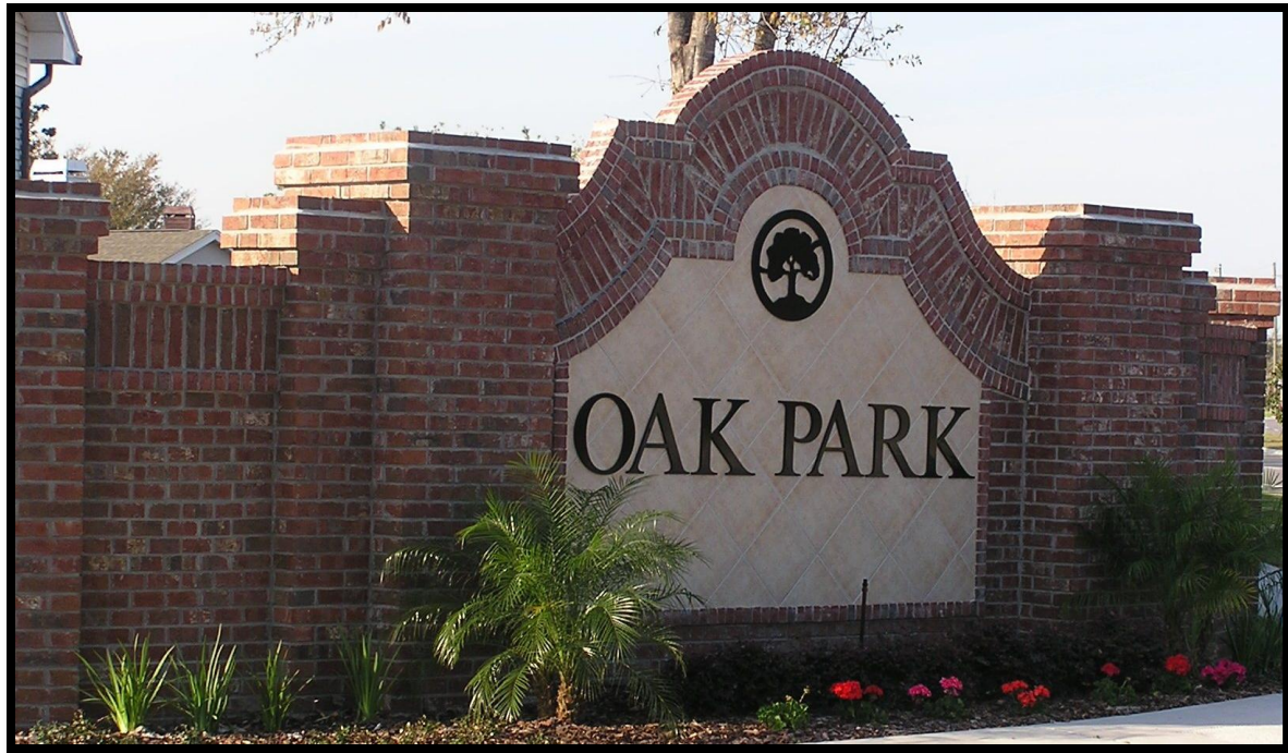
OAK PARK AFTER WALL RECONSTRUCTION
