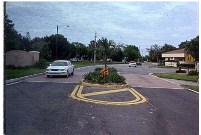
City of Orlando Center Island
