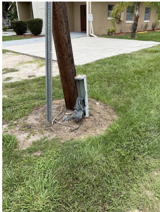
Figure 12 – Broken CenturyLink Ped Ford Dr
