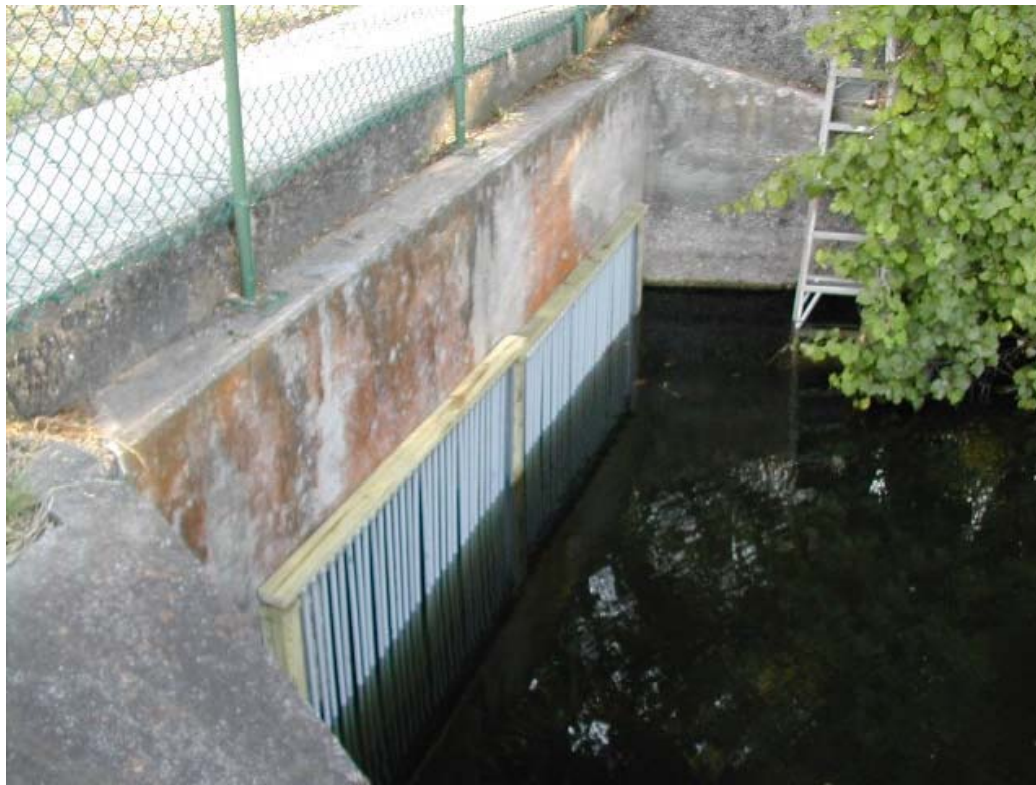
Triploid Grass Carp Barrier Installed May 2009
