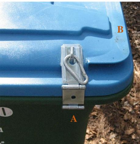
3. Lay the hinge over the lid to mark the best position for the eye of the hasp. Make sure the hinge can be locked and unlocked easily. Pre-drill 3/16" holes in the marked spots on the lid of the can for the hasp eye.
