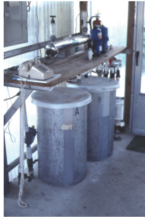
Figure 3. Fertilizer stock tanks for rockwool or perlite systems located under proportioner bench.
