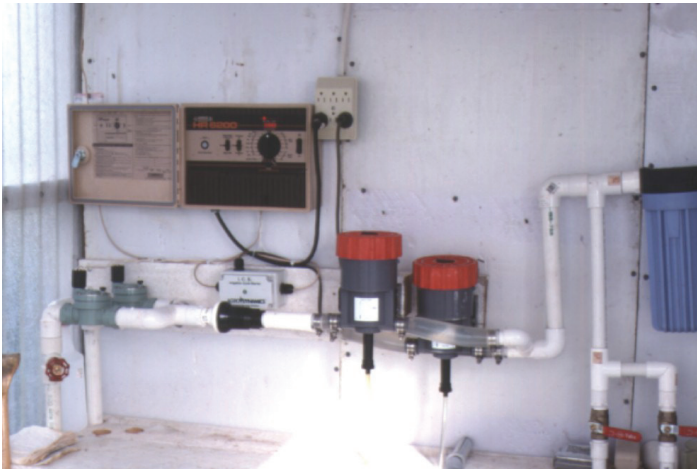
Figure 4. Irrigation controller, solenoid valves, pressure regulator, and proportioners for rockwool or perlite systems.
