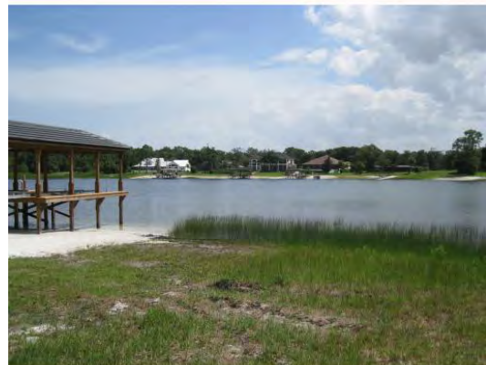
Figure 9. Shore erosion in Lake Mary
