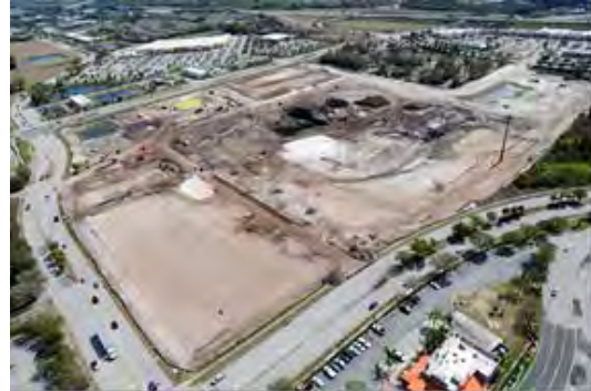
The correct way to prepare a property for development.
