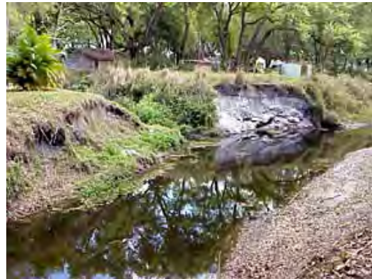
Area along the Little Wekiva River Basin where soil erosion is visible.
