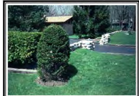
This low floodwall has landscaping to minimize the adverse impact on the property's appearance.
