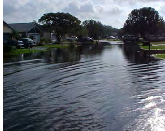
Figure 10. Proper Stormwater Management
