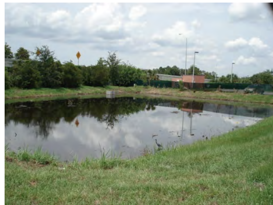
Storm retention pond in the City of Longwood.
