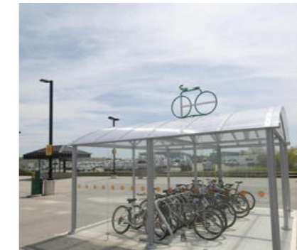
Basic sheltered bicycle parking provides security and weather protection.
