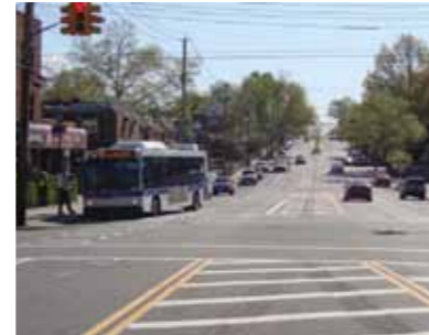
Allerton Avenue in New York City added a median turn lane, bike lanes, and wide parking lanes.
